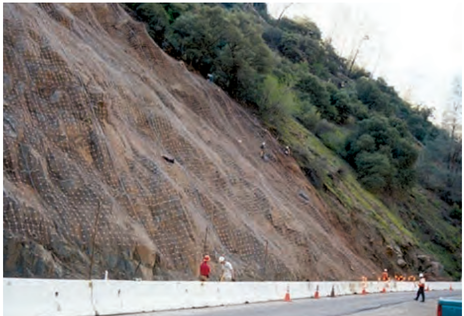
Figure C21. Example of wire mesh placed over a rocky slope to contain the rocks that may come down.
